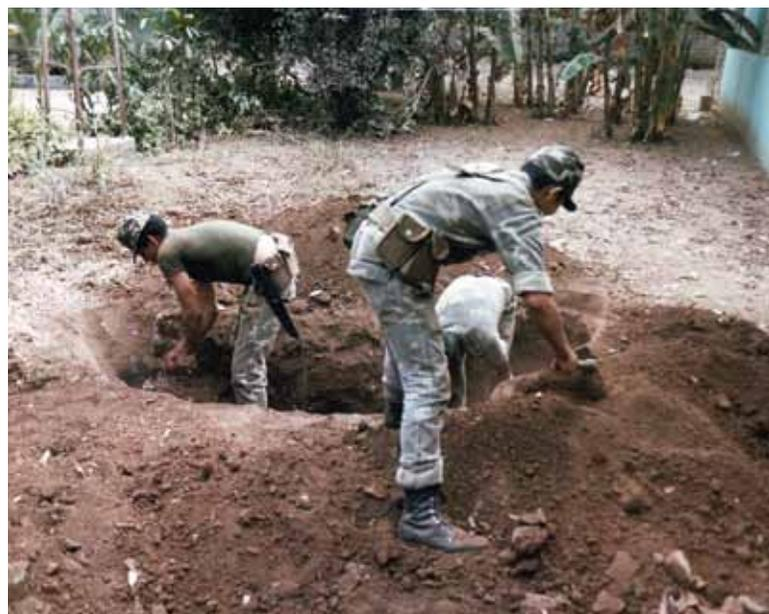
*The primary digging tool for the ground defensive positions was the U.S. Army folding entrenching tool. The rock-hard dirt was used to fill the sandbag barriers in front of each position.*
